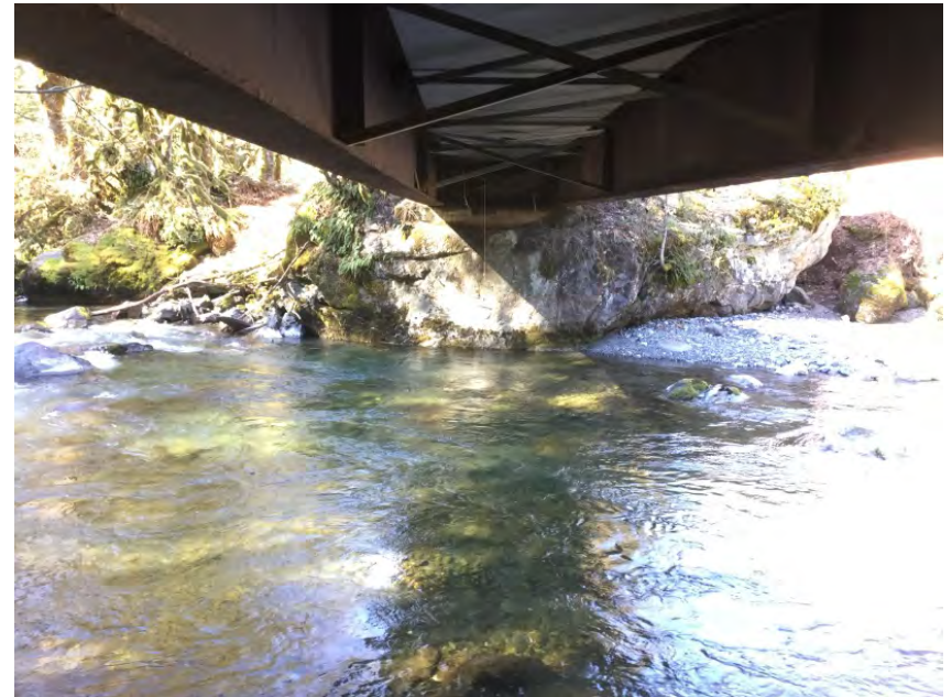
Left Bank Abutment when facing downstream
