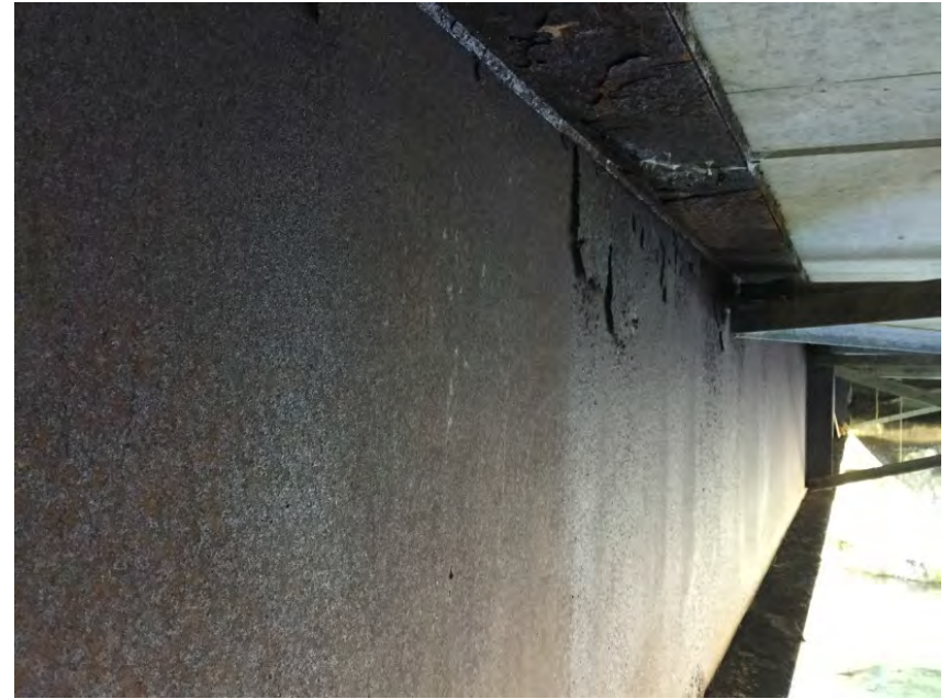
Steel delamination
