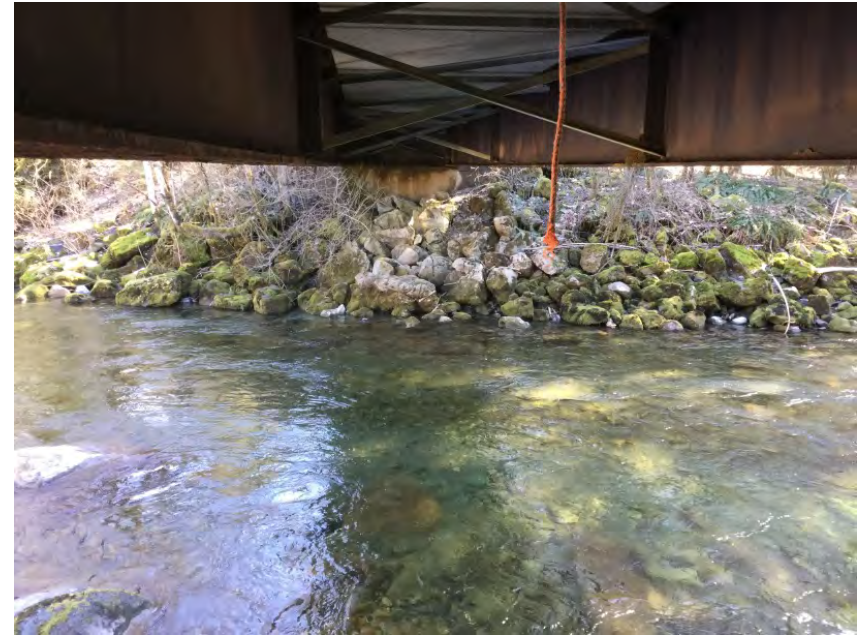
Right Bank Abutment when facing downstream
